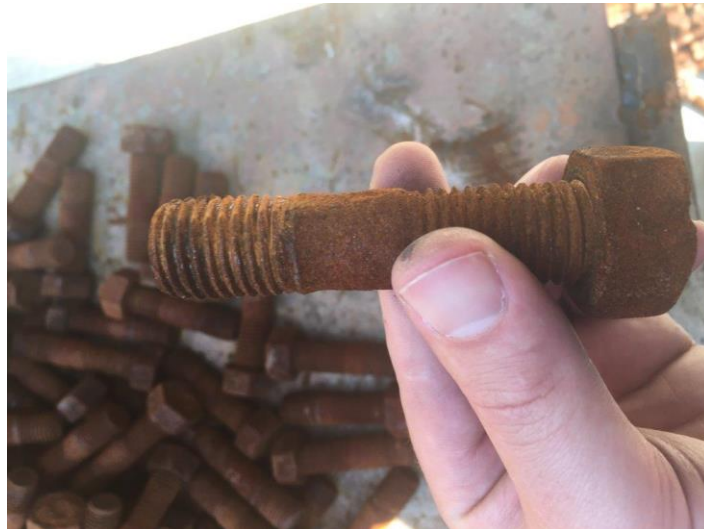
Figure 6: Corrosion of carbon steel bolt.
